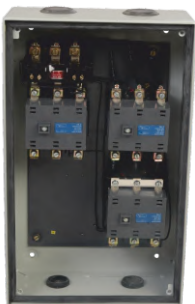
Interior View of ML SASD
